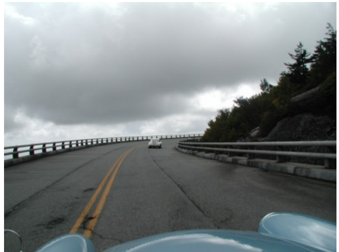
The Linn Cove Viaduct on the Blue Ridge Parkway. (Picture taken from Danny Jacob's MGA)
